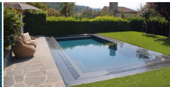
STONE COVERED OVERFLOW CHANNEL
